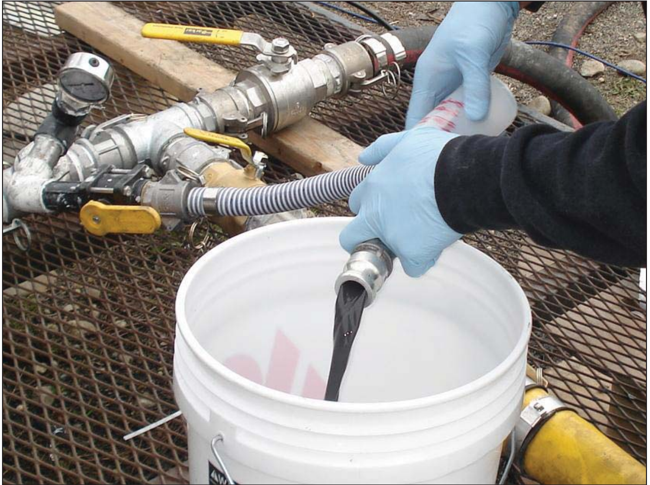
Figure 5-18. Picture of ZVI injection solution during injection.
