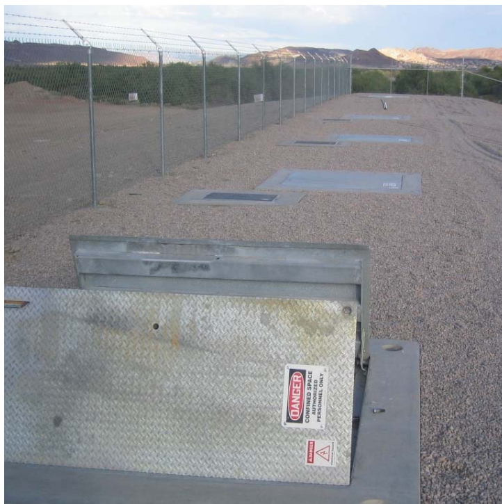
Figure A-18. Injection well vaults. (NDEP AMPAC Case File)
