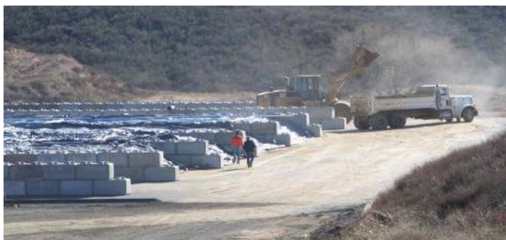
Figure 8-7. Cement-lined treatment cells. (Courtesy CDM Corp.)
