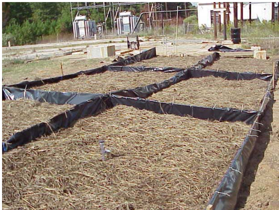
Figure 8-4. Soil treatment pilot cells at Longhorn Army Ammunition Plant. (Source: Nzengung, Das, and Kastner 2001)
