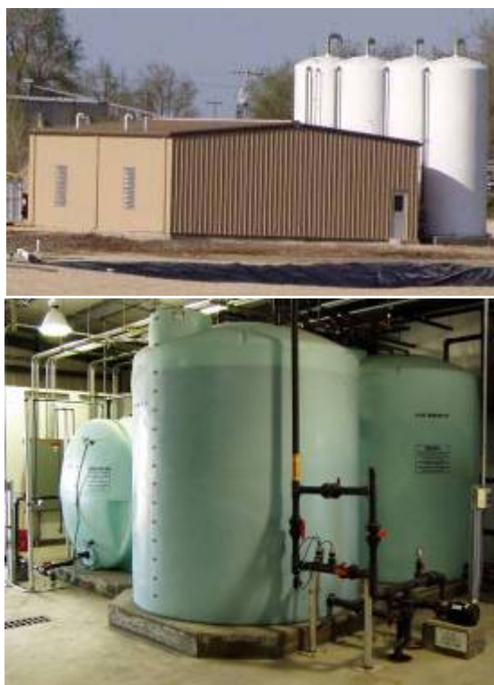
Figure 7-8. Pyrodex biodegradation system.
