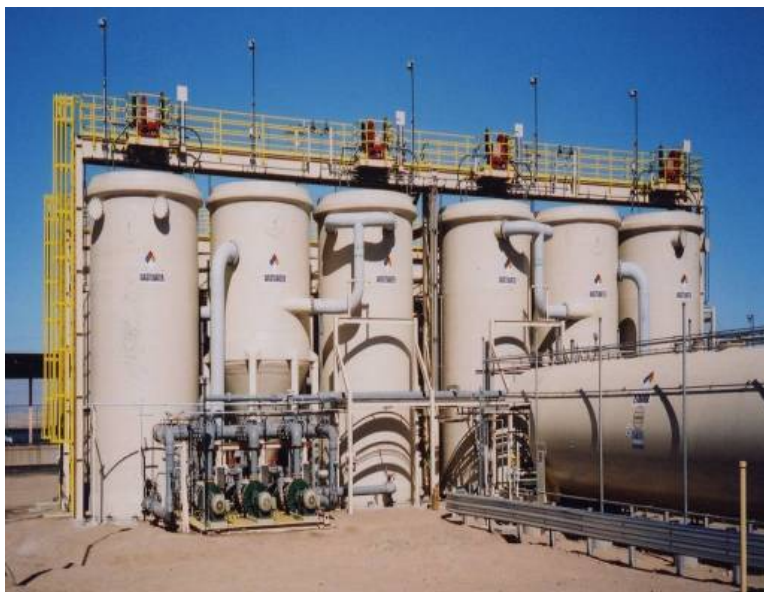
Figure 7-5. Kerr-McGee (Tronox) FBR System.
