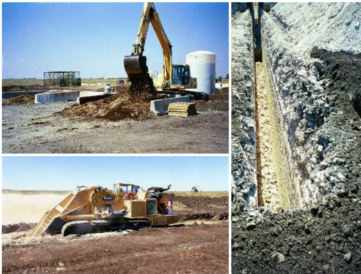
Figure A-30. Area S trench construction: the mixing area (above left), rock trencher in operation (below left), and top view of trench results (right).
