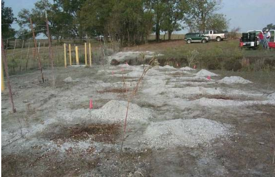
Figure A-34. Bioboring row after completion.
