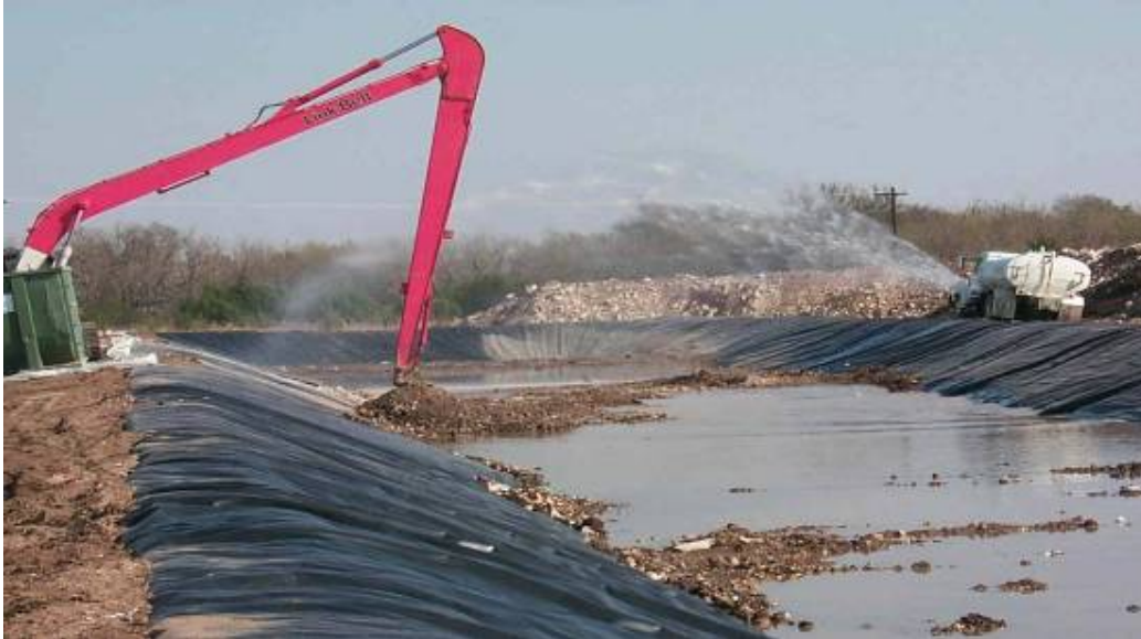
Figure A-38. Soil treatment cell construction at Area M.
