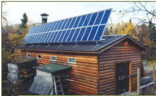
An off-grid PV system at Brooks Camp, AK, powered an air sparging pump that operated only during daylight hours, which sufficiently treated contaminated groundwater while avoiding energy loss and freeze potential associated with battery storage.
