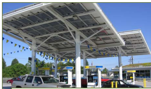
Sustainable redevelopment of a remediated brownfield site formerly used as a gasoline station in Eugene, OR, focused on building a biofuel station with solar power along with low impact development elements such as bioswales; the biofuel is made of discarded cooking oil collected across the state.
