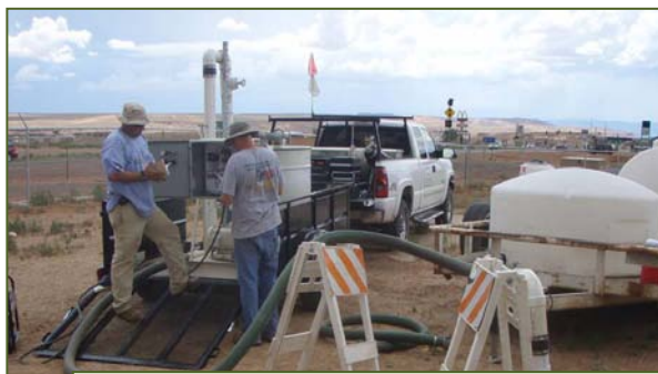
EPA Region 9 investigation of LUST-contaminated soil and groundwater affecting Navajo Nation and Hopi Tribe tribal lands near Tuba City, AZ, involved use of a conceptual site model and mobile laboratory to guide subsurface application of food-grade vegetable oil that accelerated bioremediation of contaminated soil.
