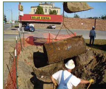
Surgical excavation and tank removal at the G&L Clothing site in Illinois allowed for minimal site disturbance and maximum recycling or reuse of excavated materials.
