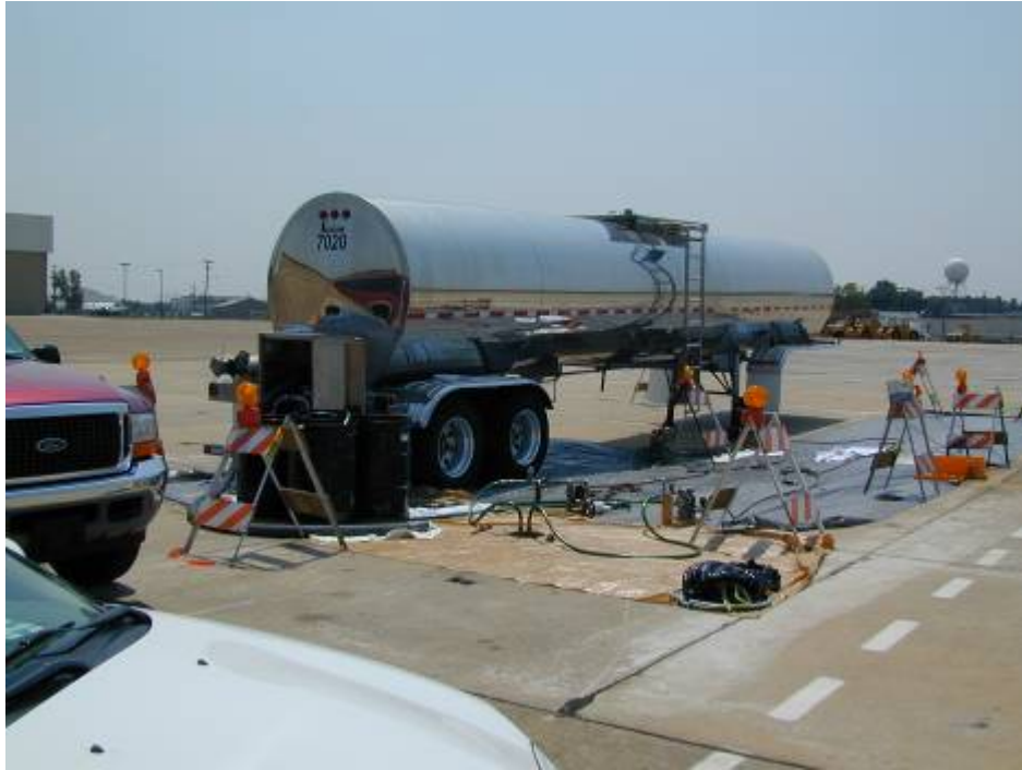
Figure 5.3 Typical Injection System Layout for Pure Edible Oil, Naval Support Activity Mid-South, Tennessee
