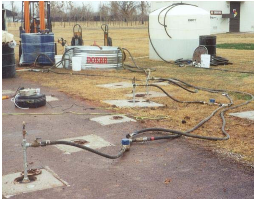
Figure 1.8 Typical Oil Emulsion Injection System Layout
