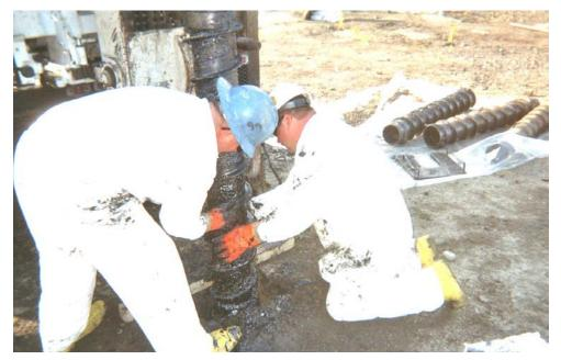
Auger Flight Coated with Viscous Coal Tar, 10/03
