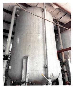
Picture 2. Granular activated carbon unit (20,000 pound)
