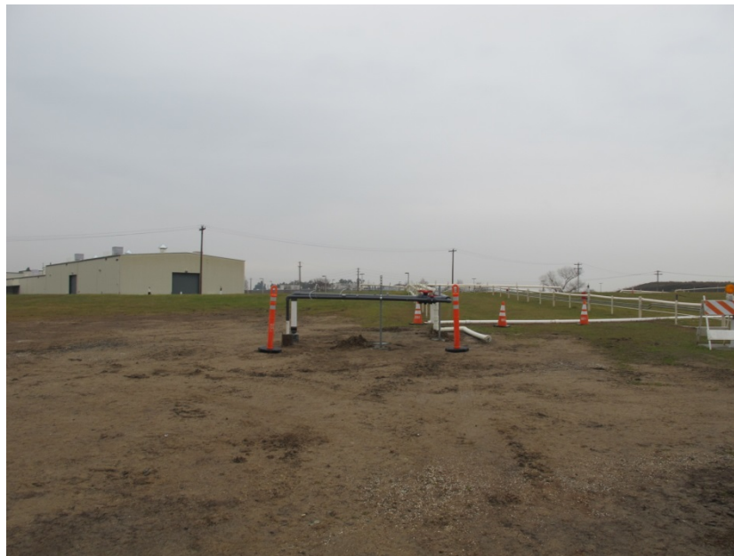
Photo 8. Site after cap restoration.
