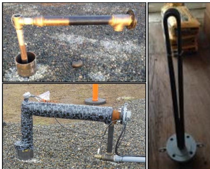
Figure 5.4.4. Injection Wellheads
