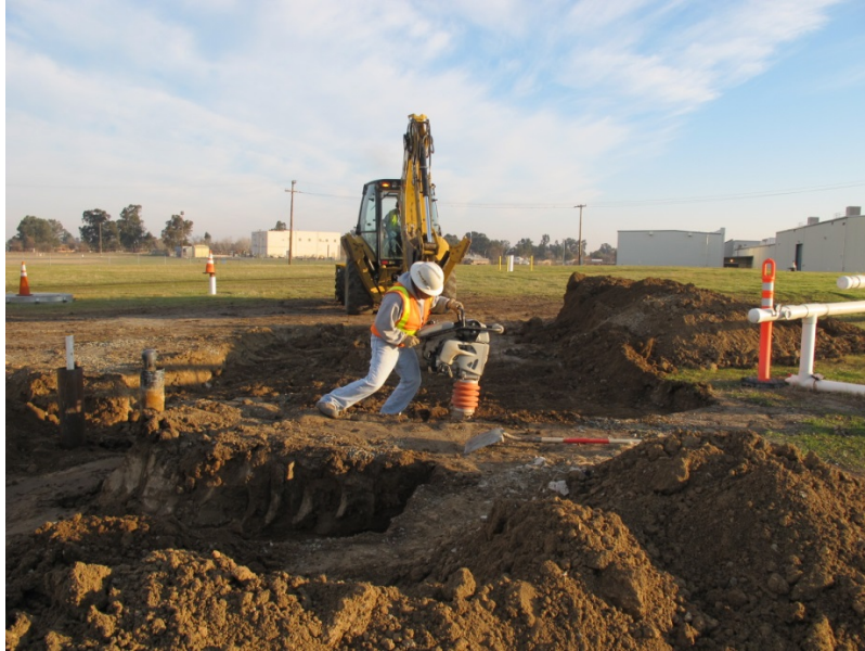
Photo 7. Backfill and compaction.
