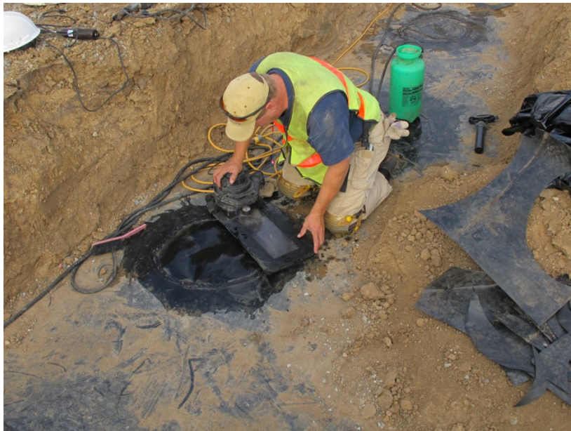
Photo 4. Vacuum Test on a patch.
