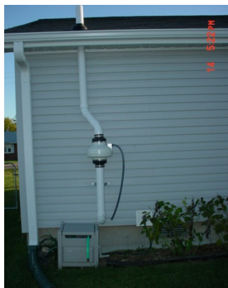
Figure J-3. Active SSD system.
