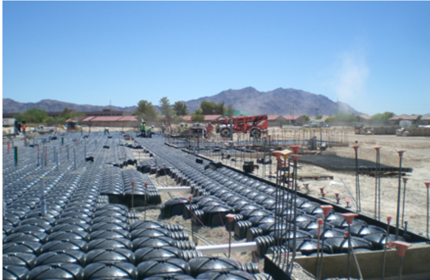
Figure J-4. Cupolex aerated floor system.
