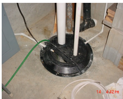
Figure J-2. Passive sump mitigation system.
