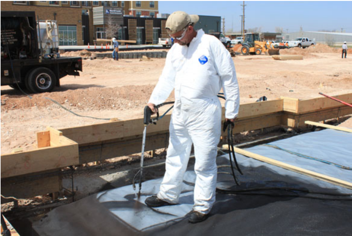
Figure J-1 Spray-applied membrane.
