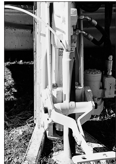
Figure 4.31. A grout machine and flexible tubing allow bottom-up grouting as the outer casing is retrieved.
