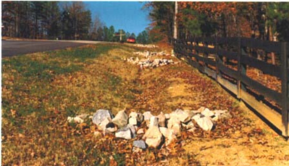
Figure 3-11. Riprap check dams installed in a roadside swale. (Source: ERDC-CERL, 2004)
