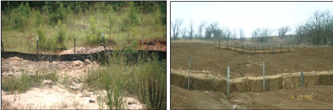
Figure 3-22. Silt fence and straw bale sediment barriers. (Source: ERDC-CERL, 2004)
