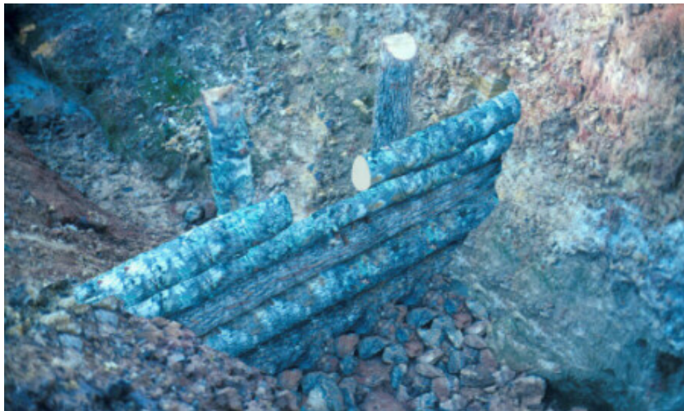
Figure 3-13. Log check dam. (Source: ERDC-CERL, 2004)
