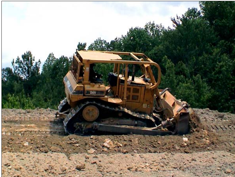
Figure 3-24. Berm slope grading.
