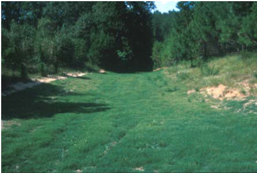
Figure 3-1. Grass-lined swale. (Source: ERDC-CERL, 2004)
