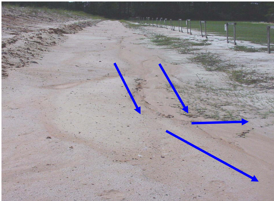
Figure 2-4. Swale showing sediment transport.
