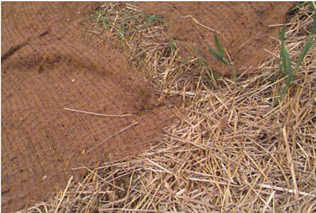
Figure 3-6. Erosion control mat and hay mulch. (Source: ERDC-CERL, 2004)
