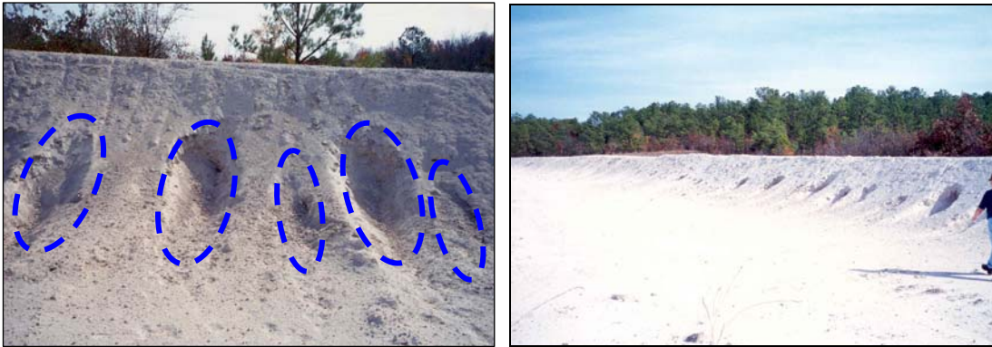
Figure 3-25. Typical 25-meter range impact berm and bullet pockets.
