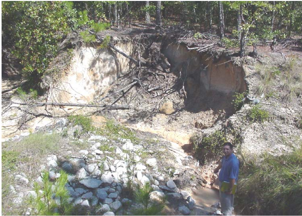
Figure 2-7. Intermittent stream bank instability.
