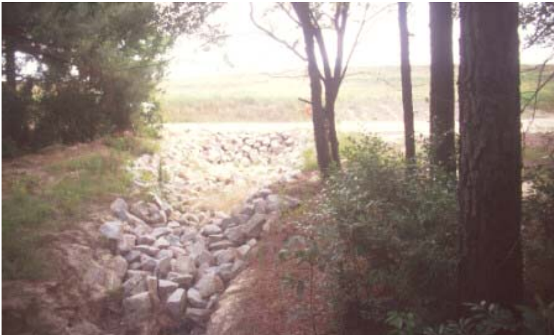
Figure 3-16. Riprap-lined channel. (Source: ERDC-CERL, 2004)
