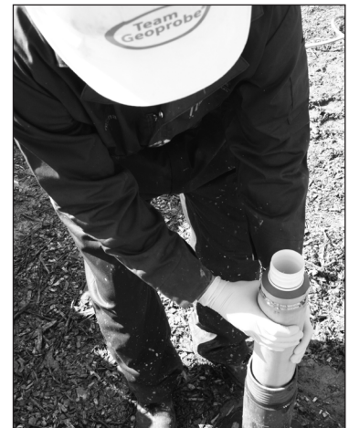
Figure 4.23. Geoprobe® prepacked screens may be installed through the outer casing when an expendable cutting shoe is used.
