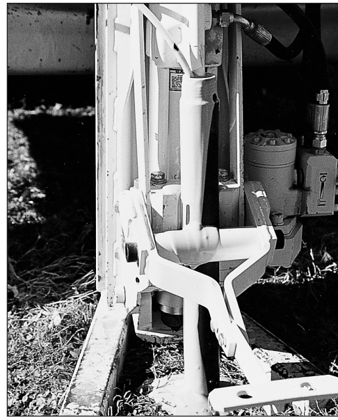
Figure 4.22. A grout machine and flexible tubing allow bottom-up grouting as the outer casing is retrieved.
